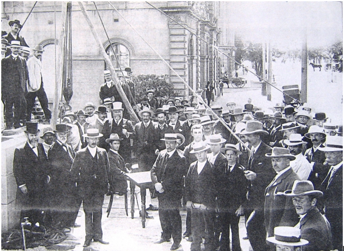
Laying of the foundation stone of New Zealand Insurance Building (now demolished) in St George's Terrace, 10 January 1905. Forward of the seated gentleman at the table, Talbot Hobbs is to the left and Dean Smith to the right (in boater hats), with John Forrest, in pale coloured top hat behind ( Western Mail , 28 January 1905, p.27).
